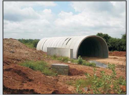
✓ Bangalore Mysore Infrastructure Corridor Project, India Structures consisting of culverts, cattle pass, underpass and Minor bridges
