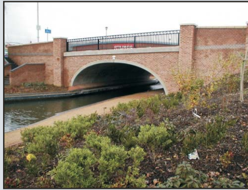
✓ Shrub Hill Canal Bridge - Worcester, UK
