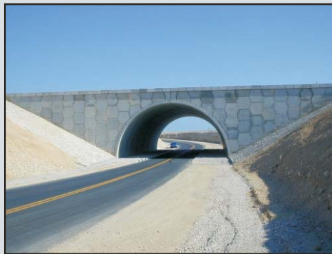
✓ Vehicle Underpass, UAE
